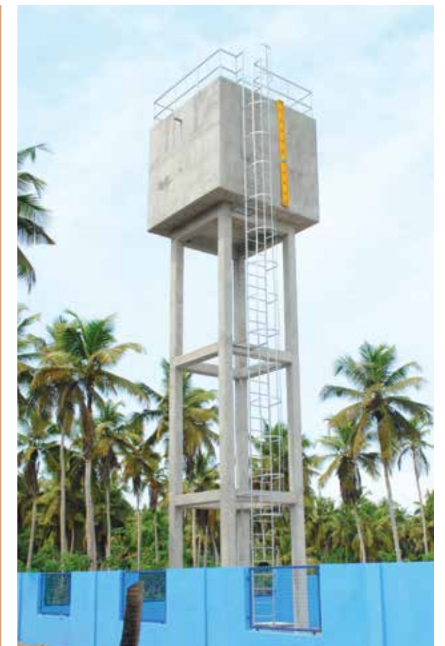
Water treatment, pumping and storage plant constructed by Kosmos Energy.
