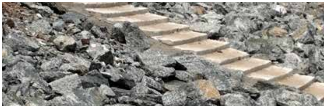
Picture 10: Stone pitching overlay for the Keyime Dam wall
