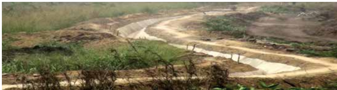
Picture 9: Dam canals through which water flows to farmlands for irrigation purposes
