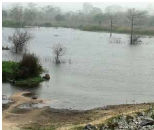
Picture 11: The Keyime Dam Source: Field Survey, 2016
