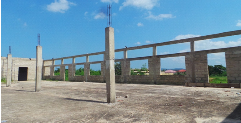
Picture 16: A section of the uncompleted assembly hall/dining hall complex
