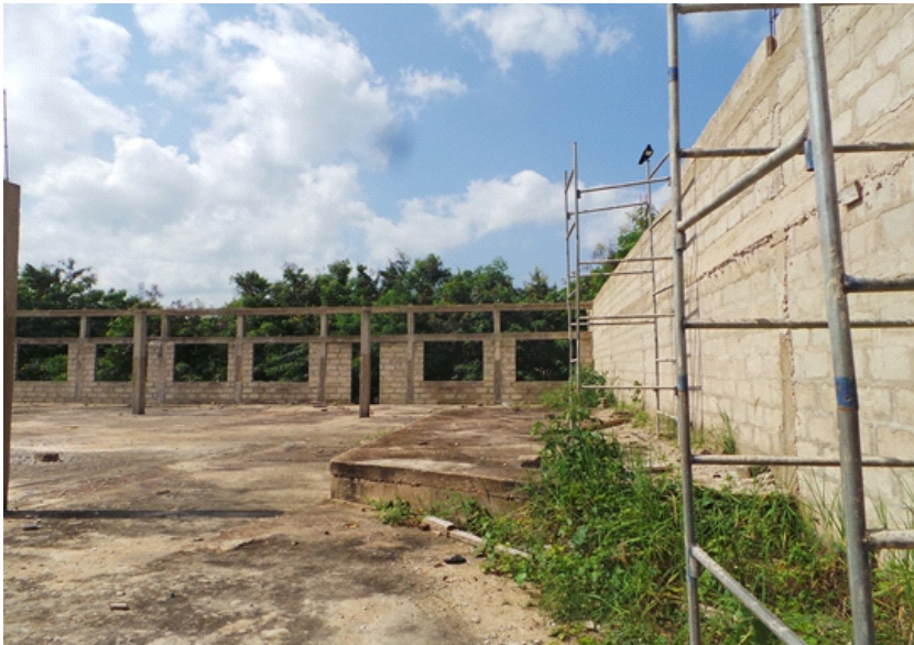
Picture 17: Another section of the uncompleted assembly/dining hall
