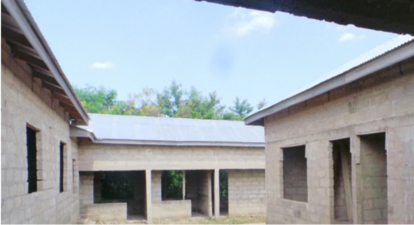
Picture 18: Kitchen section of project still in its construction phase
