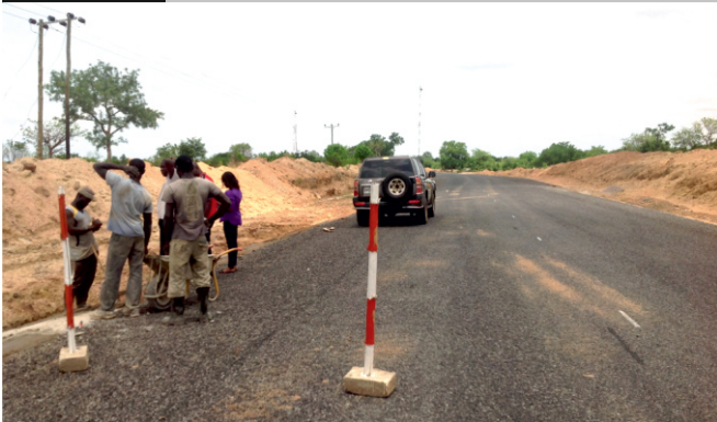
Workers on the Navrongo - Tumu Road
