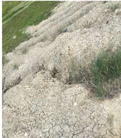
Picture 10: Gully erosion on the downstream slope of the dam
