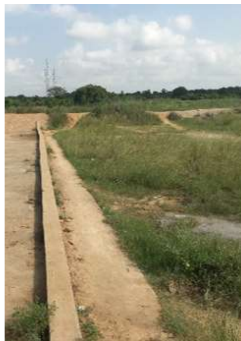
Picture 6: Dam Overflow
