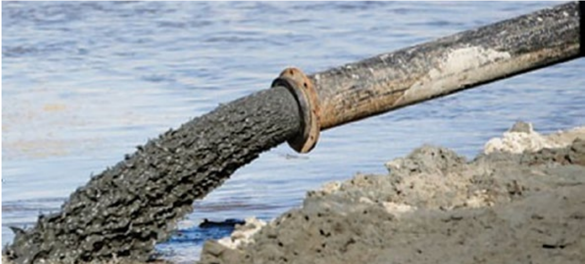
Picture 3: Slurry Pipeline Waste Disposal
